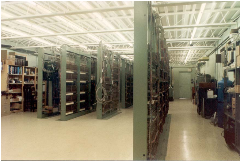
The S.A.-1 Community Crossbar Equipment could accommodate 480 telephone lines and 1500 terminals
